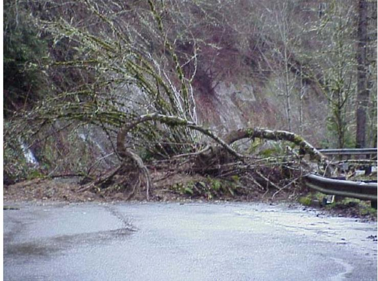
**Alternative 3:** Debris clearing and rock scaling of the slide area. This is expected to cost \$75,000 the first time, and require \$50,000 repeated “treatments” every 5 years. After clearing/scaling, slides are expected to occur much less frequently, once every 4 years on average. The benefits are having much less frequent repair and traffic routing costs. This approach has been used successfully by ODOT (according to Scott Bryan)
